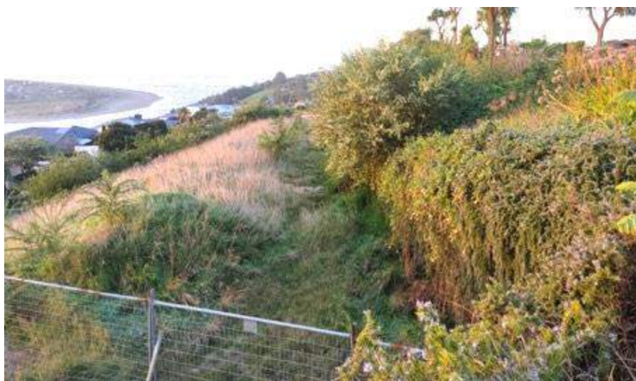
Figure 11: View of the retaining wall west of Lot 7, looking northeast (Area 1)
