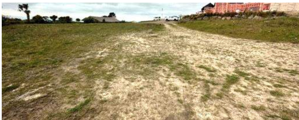
Figure 10: View of the car park area (Lots 5 - 7), looking southeast (Area 1)
