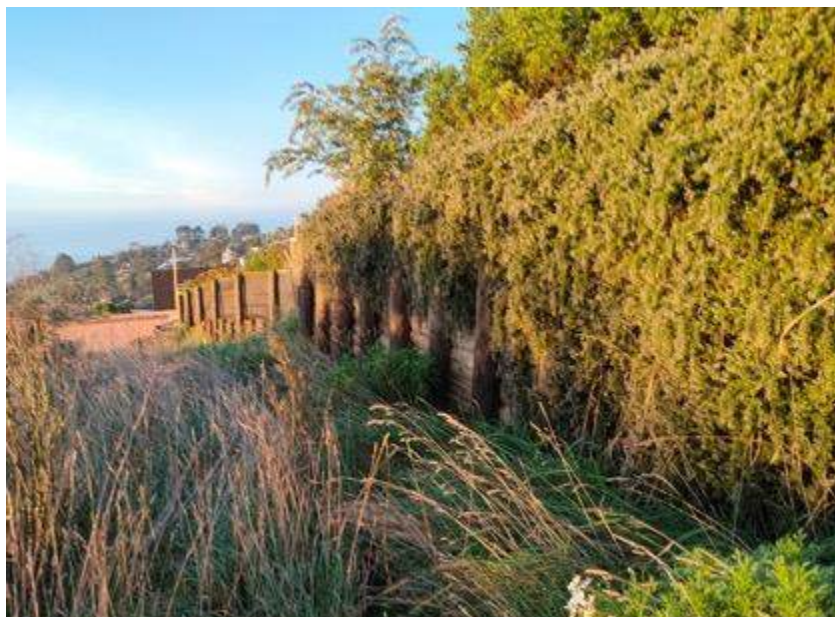
Figure 12: View of the retaining wall below Lot 7, looking northeast (Area 1)
